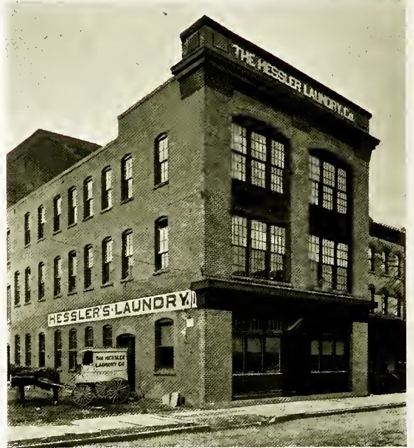
Hessler Laundry Co. Plant East South Street
